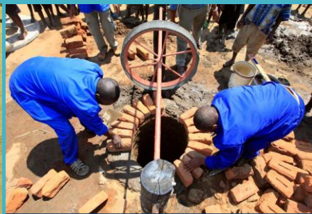
Pump installation process
