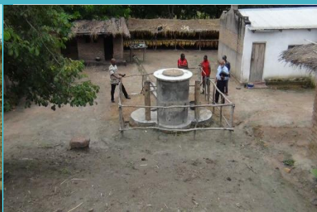
Pump installation process
