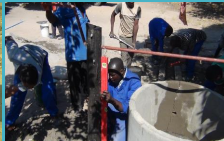
Pump installation process
