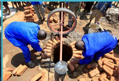
Pump installation progress
